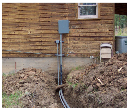
New Electrical Feed to McBride
